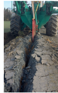
Installation of a high-pressure gas pipeline using the plowing technique
