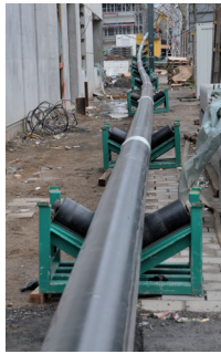
Installation of a gas pipeline with multi-layer coating system using the flush-drilling technique
