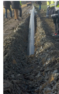
Installation of a high-pressure gas pipeline using the plowing technique
