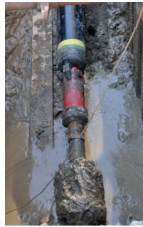
Installation of a gas pipeline with multi-layer coating system using the flush-drilling technique
