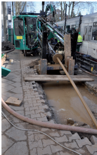
Installation of a gas pipeline with multi-layer coating system using the flush-drilling technique
