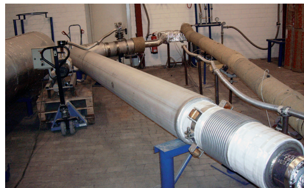
Figure 3: FW-Kammer-Pipe during assembly
